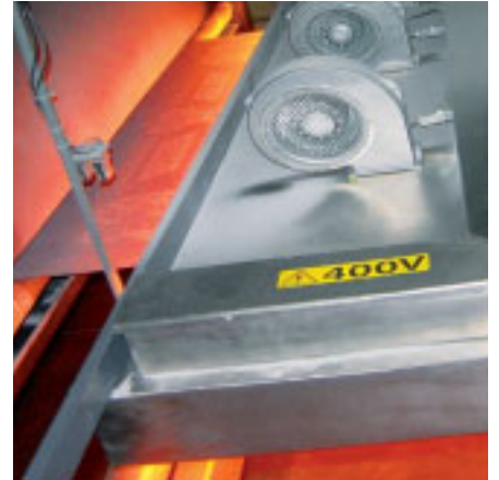
Adhesives on carpets activation before lamination
